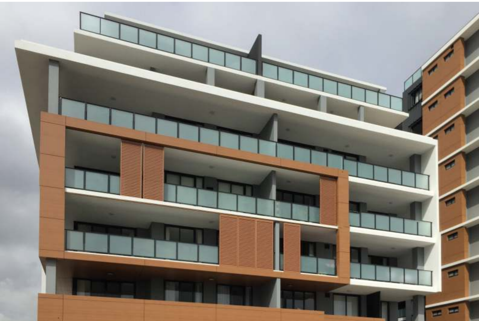
Endeavour apartments (Australia) Illusions Design Wood English Cherry Architect: Loucas Architects
